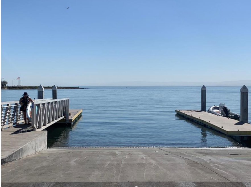
Boat launch ramp and boarding floats
