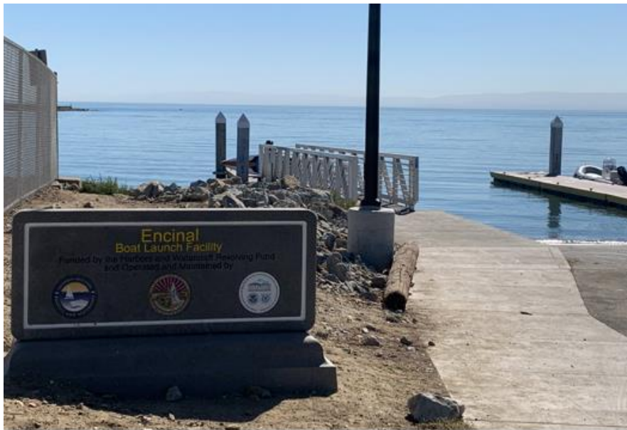
Project credit sign with boarding float in the background
